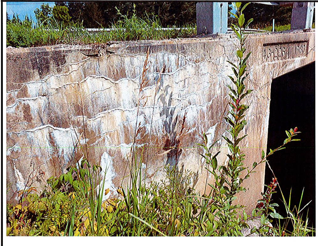
Photo 11 Horizontal and vertical cracks with efflorescence and small spall on SW wingwall
