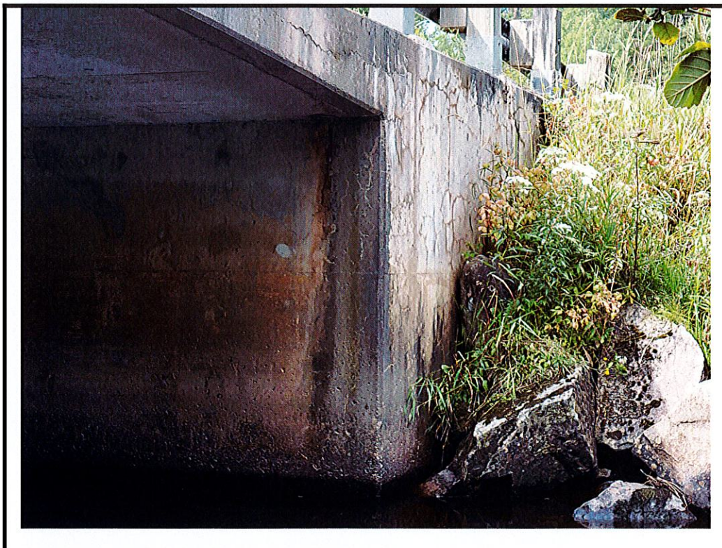
Photo 14 Narrow map cracks on SE wingwall
