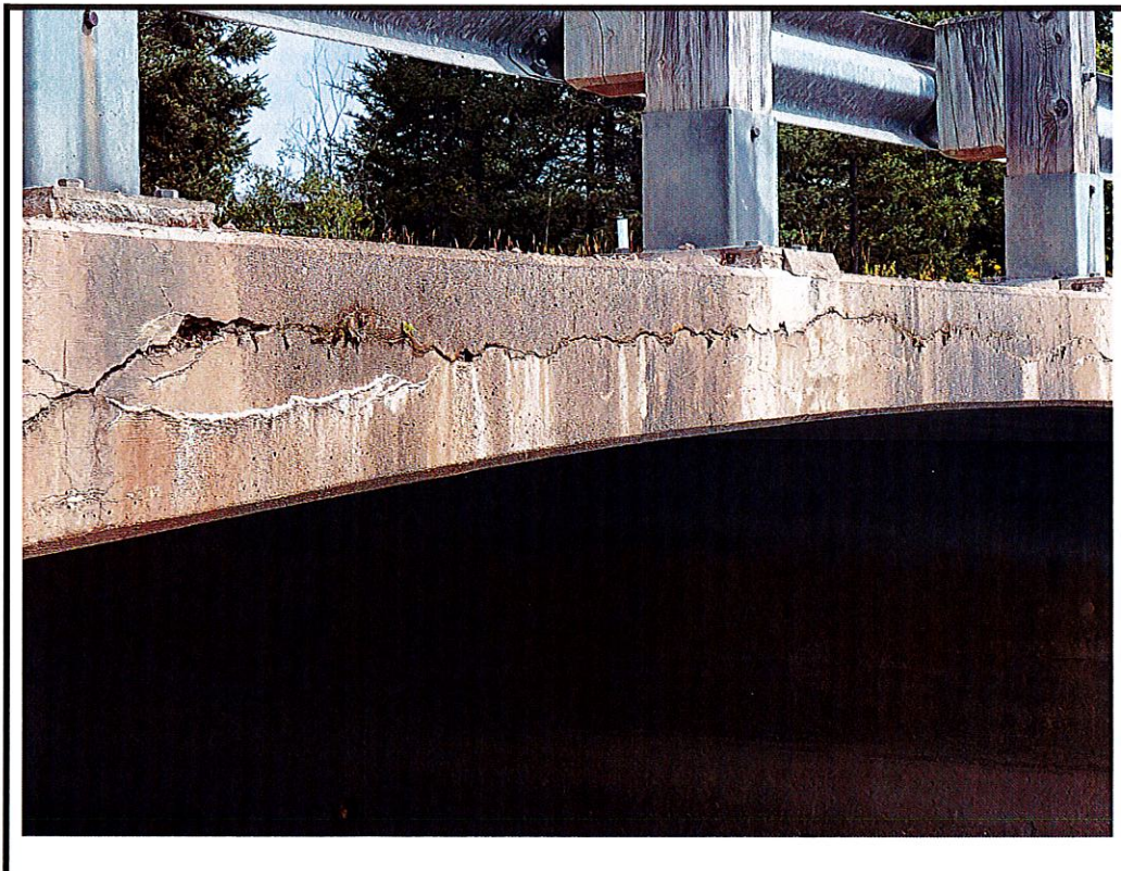
Photo 12 Wide horizontal cracks with efflorescence on south exterior soffit
