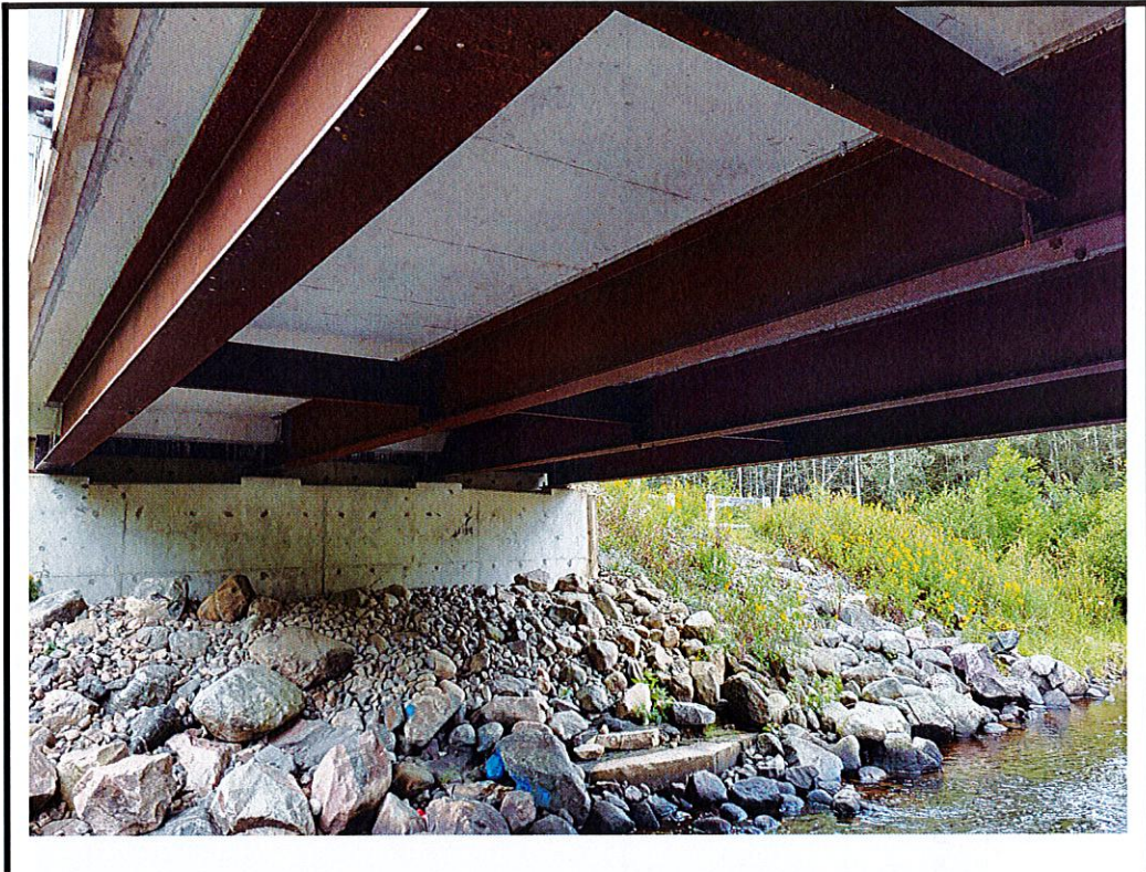
Photo 13 Typical underside of structure (girders, diaphragms, and soffit)
