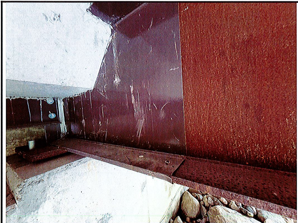
Photo 12 Localized coating failure (delamination) on girder ends
