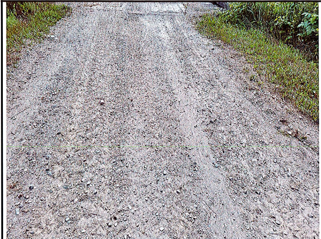
Photo 7 Loose gravel, tire rutting & potholes at ends of deck on approach wearing surface
