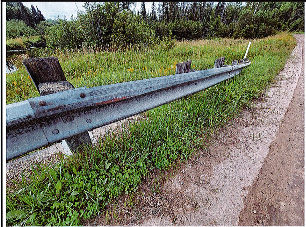
Photo 9 Dents, abrasions, and substandard end treatment on NW approach guide rail
