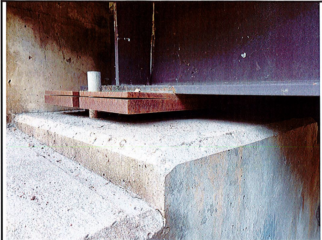
Photo 11 Minor deformation and light corrosion on steel bearing plate, NE bearing
