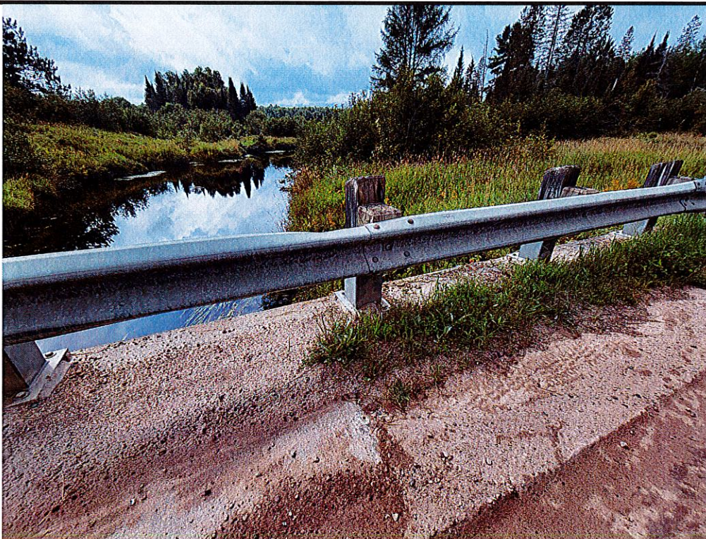
Photo 8 Deformed steel beam deck barrier on north edge of deck
