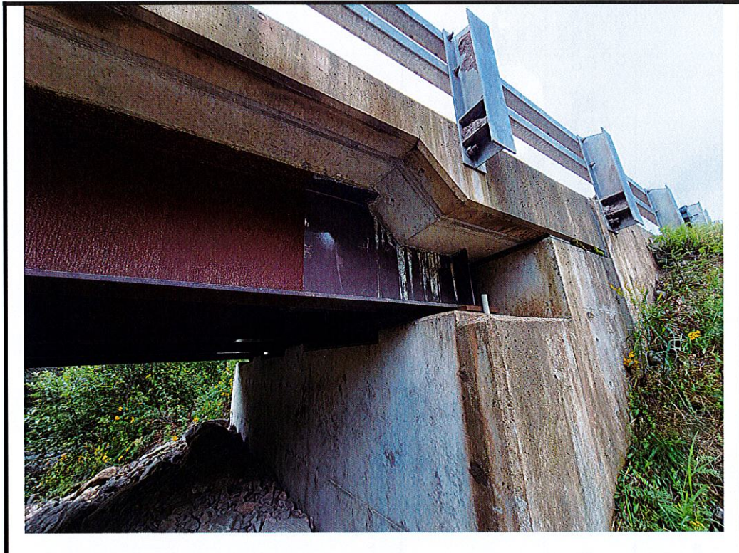
Photo 14 Damp staining on exterior soffit and wingwall SE corner of structure
