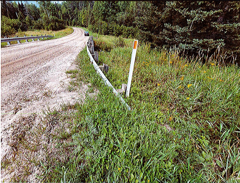
Photo 7 Substandard end treatment at south east approach barrier
