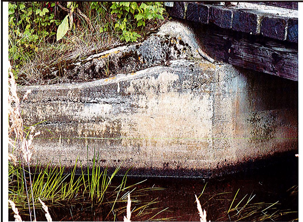
Photo 11 Moderate honeycombing and scaling noted on NW wingwall
