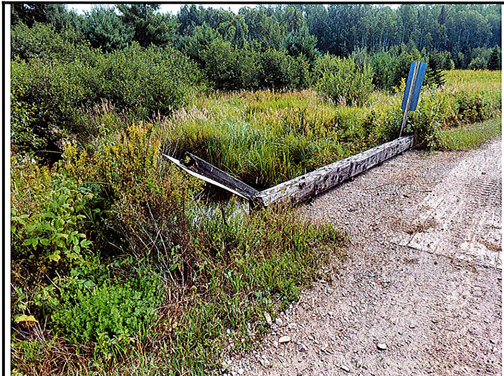
Photo 8 Hazard sign leaning away from roadway on NE corner of deck
