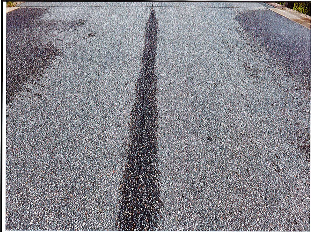
Photo 9 Wide longitudinal center-line crack on deck wearing surface
