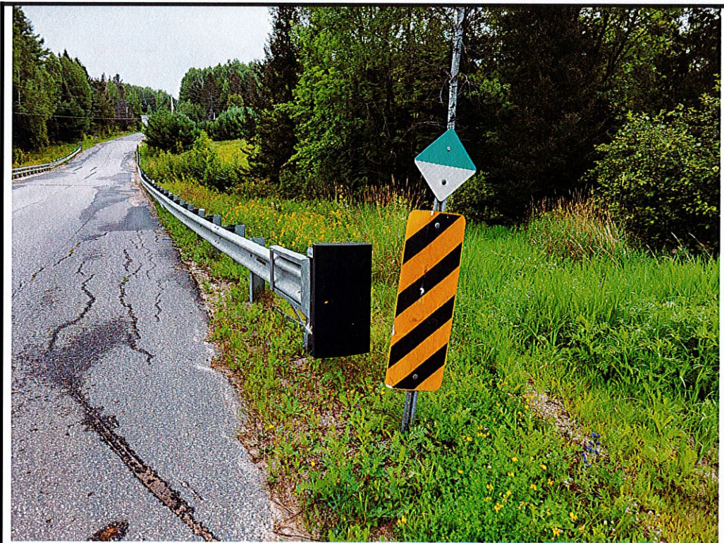
Photo 10 Hazard sign at SW approach is leaning and has minor dents and abrasions
