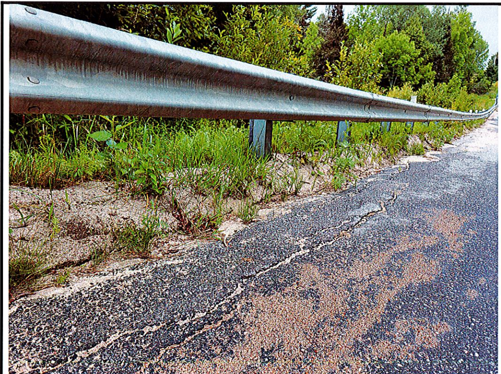
Photo 8 Accumulation of dirt and debris below approach guide rail
