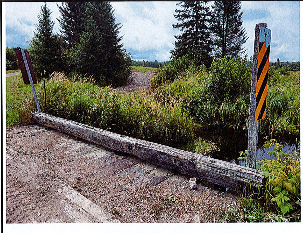
Photo 9 Rot, checks and splits on timber curb along west edge of deck
